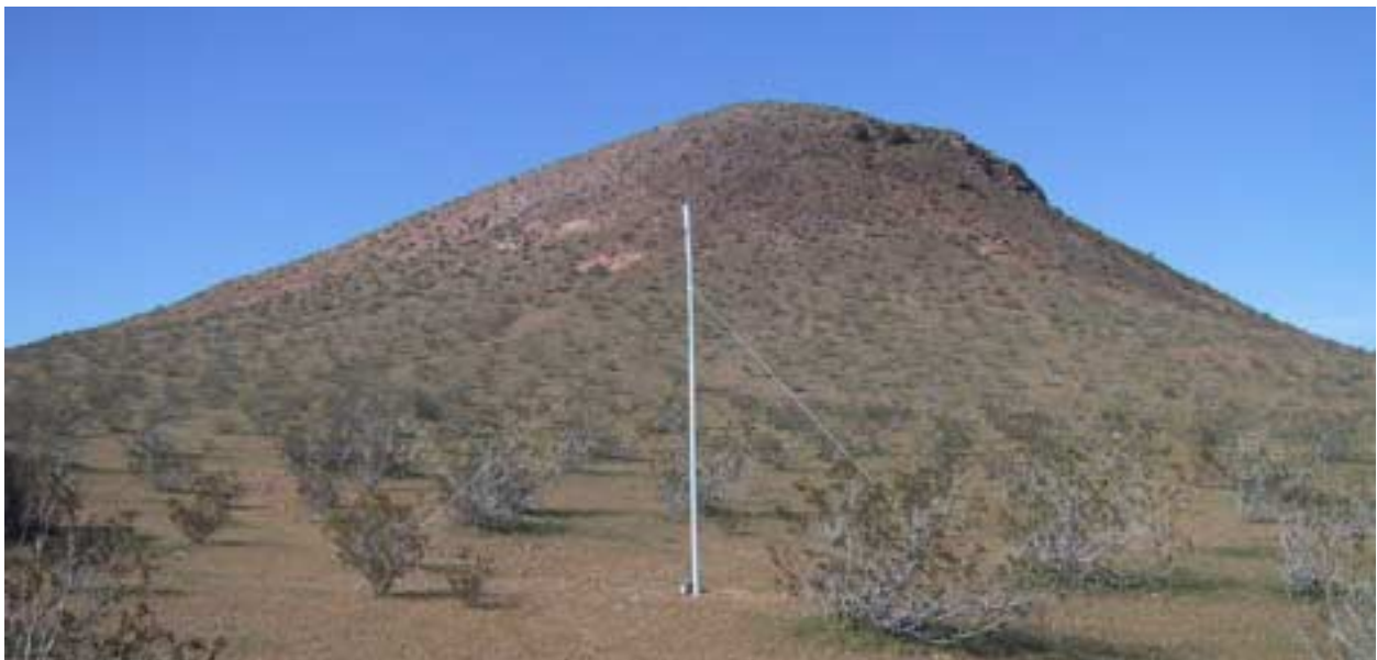
Figure 3. Installed "Backpacker" 20-Meter Test Antenna North View
