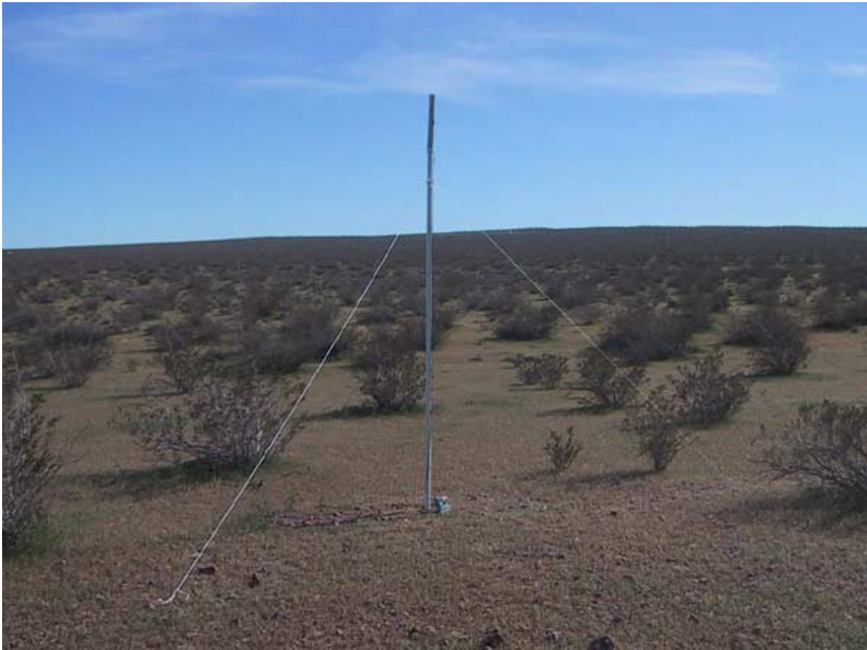
Figure 2. Installed "Backpacker" 20-Meter Test Antenna South View (Radome Installed)
